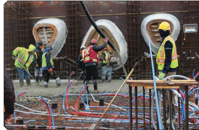
Observing proper concrete pumping procedures at ITC's Surrey Central project
